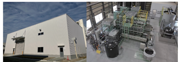
図4 リン回収棟とリン回収設備 Phosphorus recovery building and phosphorus recovery facility system
