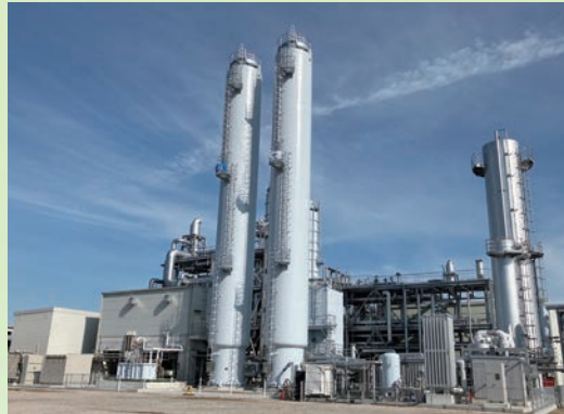
▲ The world’s first LAES commercial demonstration plant (the two tanks in the center are liquid air storage tanks)
