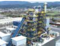
Power Plant with Circulating Fluidized Bed Boiler
