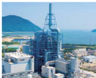
Biomass Power Generation Plant
