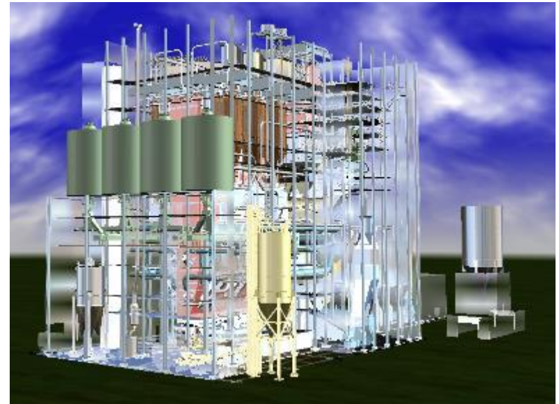
The world's largest-class 300MW dedicated biomass combustion supercritical CFB boiler (power efficiency: 40% or more)
