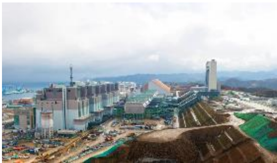
The world's first 550MW coal-biomass co-combustion ultra-supercritical CFB boiler (located at Samcheok, South Korea; started operations in 2015)
