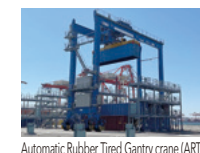
Automatic Rubber Tired Gantry crane (ARTG)
