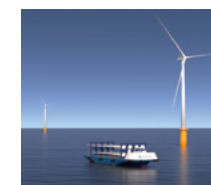
Offshore Wind Power Generation
