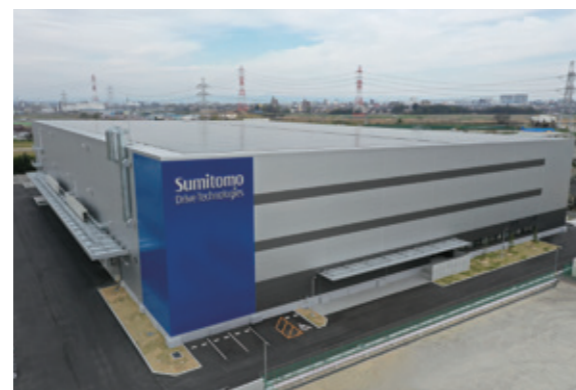
PTC Plant No. 2 (new facility in Nagoya Works)
