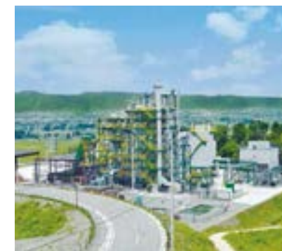
Circulating fluidized bed boiler installation
