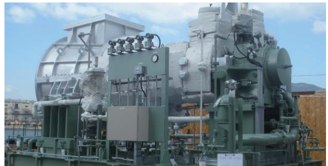
Steam turbine for power generation
