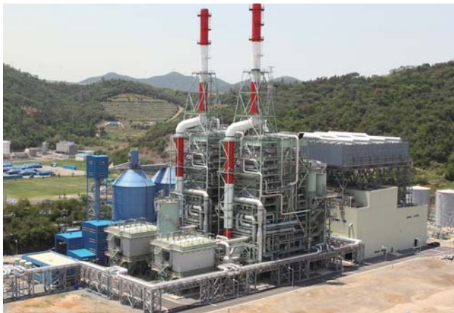
Circulating fluidized-bed (CFB) boiler
