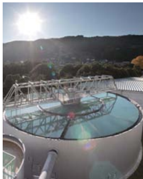
Coagulation sedimentation system "SUMI-THICKENER®"
