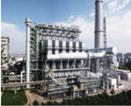
Dry activated carbon desulfurization and denitration facility
