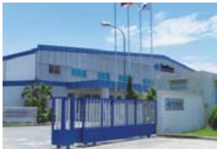
External view of motor plant (Hanoi, Vietnam)
