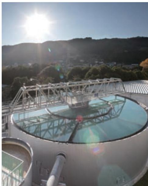
Coagulation sedimentation system "SUMI-THICKNER"
