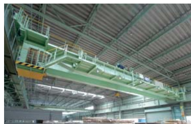
Overhead traveling crane
