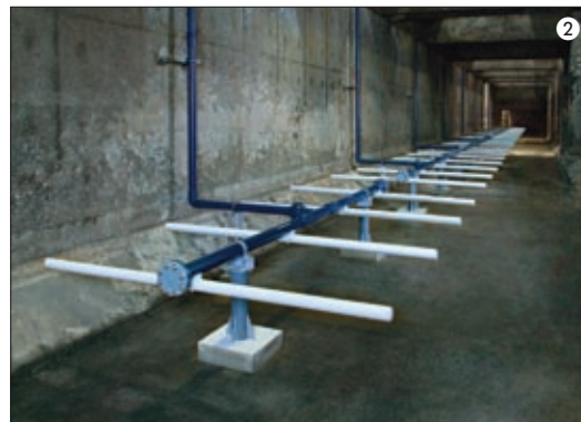
Superfine-bubble membrane tube diffuser MICRUS ®
