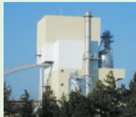
Hokuetsu Paper Mills / Kanto plant (Katsuta) Steam-generation capacity: 195t/h
