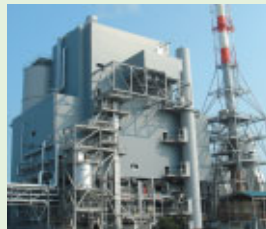
Chuetsu Pulp & Paper / Futatsuka plant Steam-generation capacity: 130t/h
