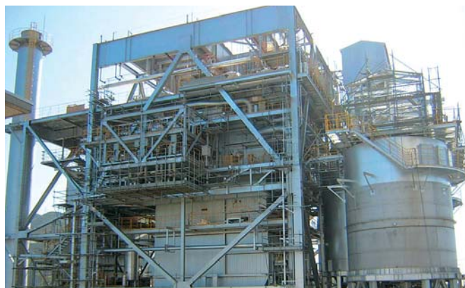
Large-scale Biomass Power Plant Facility, Summit Myojyo Power Corporation
