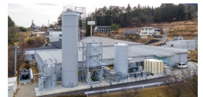
Anaerobic effluent treatment system
