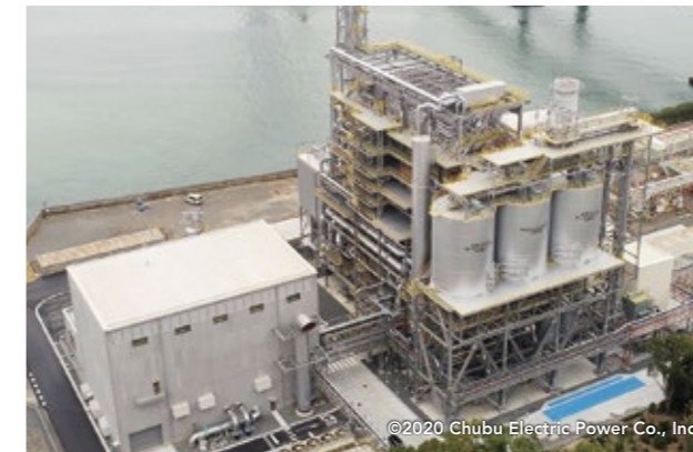
Biomass power plant (Chubu Electric Power Co., Inc.)
