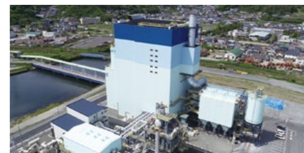
Biomass power plant (ENEOS Biomass Power Muroan G.K.)
