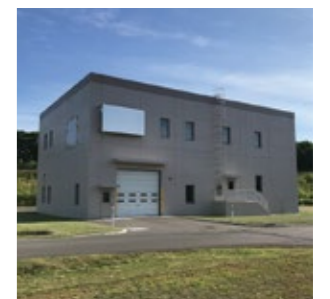
Flow control building (Iwanai/Kyowa Wastewater Management Center)
