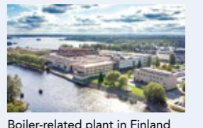
Boiler-related plant in Finland
