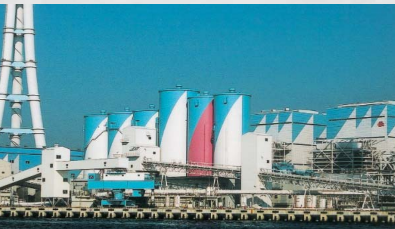
CHUBU Electric Power Co., Inc. Hekinan Power Station Ash Handling Facility
