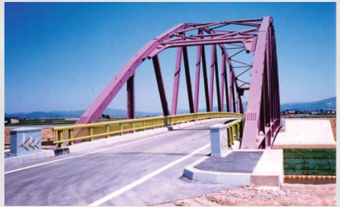
Engan-bashi Bridge (Moseushi Town, Hokkaido)
