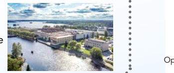
Boiler-related plant in Finland
