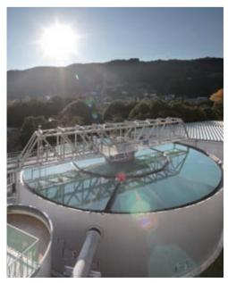
Coagulation sedimentation system "SUMI-THICKNER"
