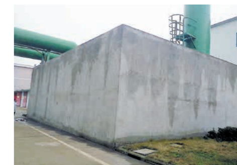
Soundproof wall at paint exhaust treatment facility
