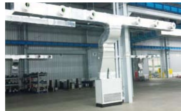
Speed reducer factory in Tangshan, China Local air-conditioning units allow rational air-conditioning use at individual work sites.
