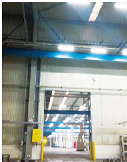
The increased number of skylights in extension to the speed reducer factory in Tangshan, China. The extension to the factory can be seen through the doorway. The number of rows of skylights has been increased from one to two.
