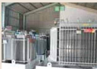
Storing transformers containing minute amount of PCB
