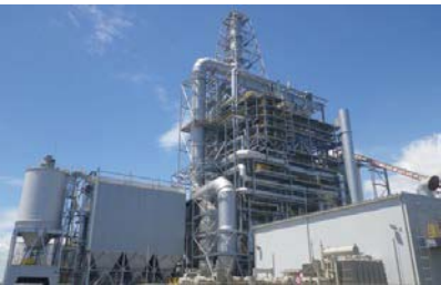
CFB Biomass Boiler (Circulating Fluidized Bed Boiler)
