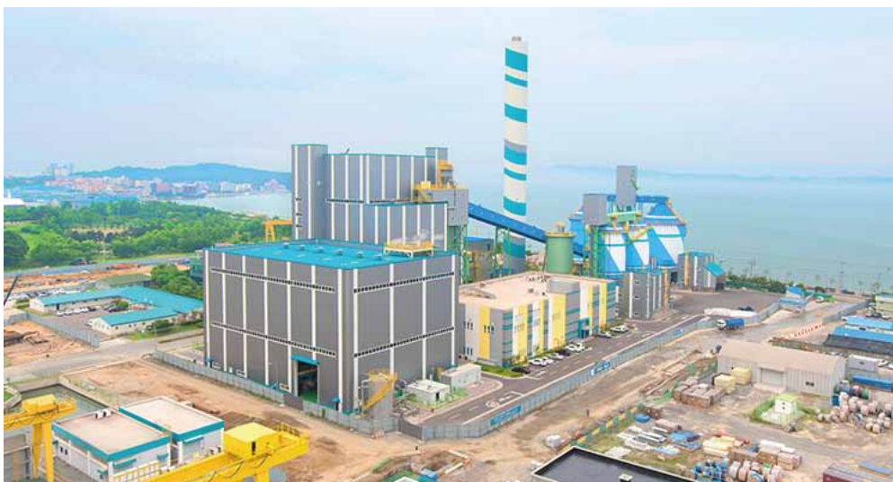
Figure 2 Dangjin Bio-1 Power Plant (105MWe, 108kg/s, 129bar(g), 540°C) produces a power of 105MWe from palm kernel shells, wood pellets, recycled wood, and sub-bituminous coal. Our CFB technology provides an ideal solution for cleanly converting biomass and low-quality coal into valuable steam and power.
