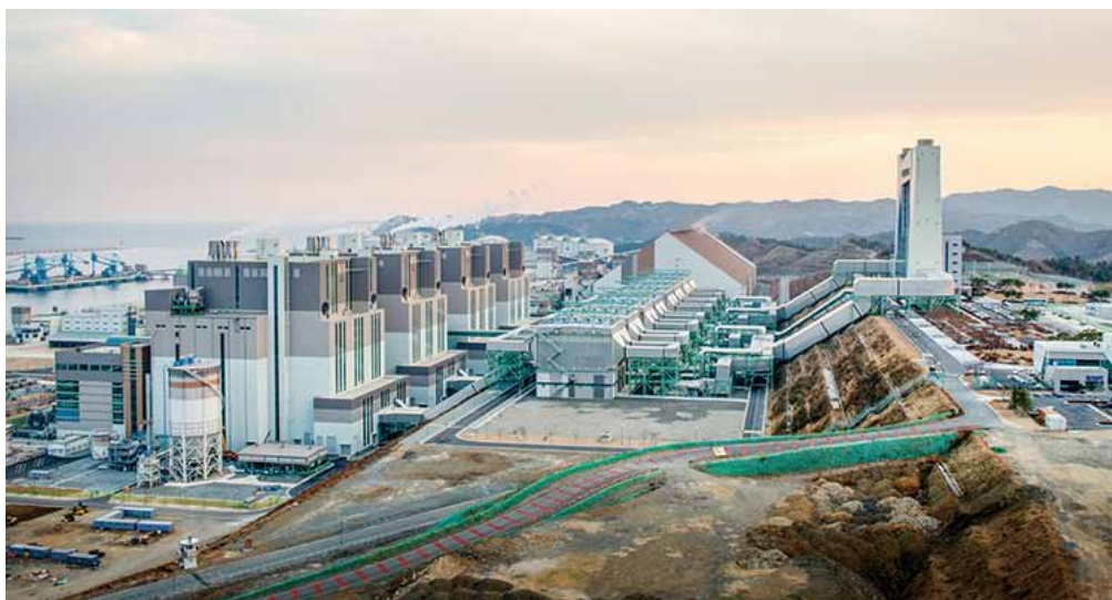
Figure 1 Massive 2.2 GW Samcheok Green Power Project (4 × 550 MWe, 437, 7/356, 4 kg/s, 257/53 bar(g), 603/603°C) in South Korea is approaching two years of full commercial operation. Utilizing the most advanced ultra-supercritical CFBs in the world, it signifies the next big step for clean and flexible power from economical solid fuels.
