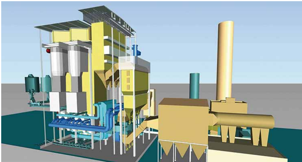
Figure 4 SFW has been awarded a contract by Tecnicas Reunidas SA and Samsung C&T EC UK to design and supply the world's largest, newly built, 100% biomass-fired 299MW CFB for Tees Renewable Energy Plant (299MWe, 229/205 kg/s, 176/43.8 bar(a), 568/568 °C) in Teesside, UK for MGT Teesside Limited.
