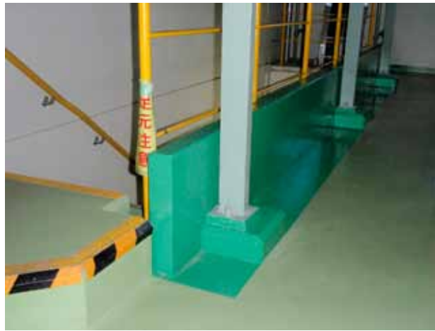
図3 防水堤 Waterproof wall
