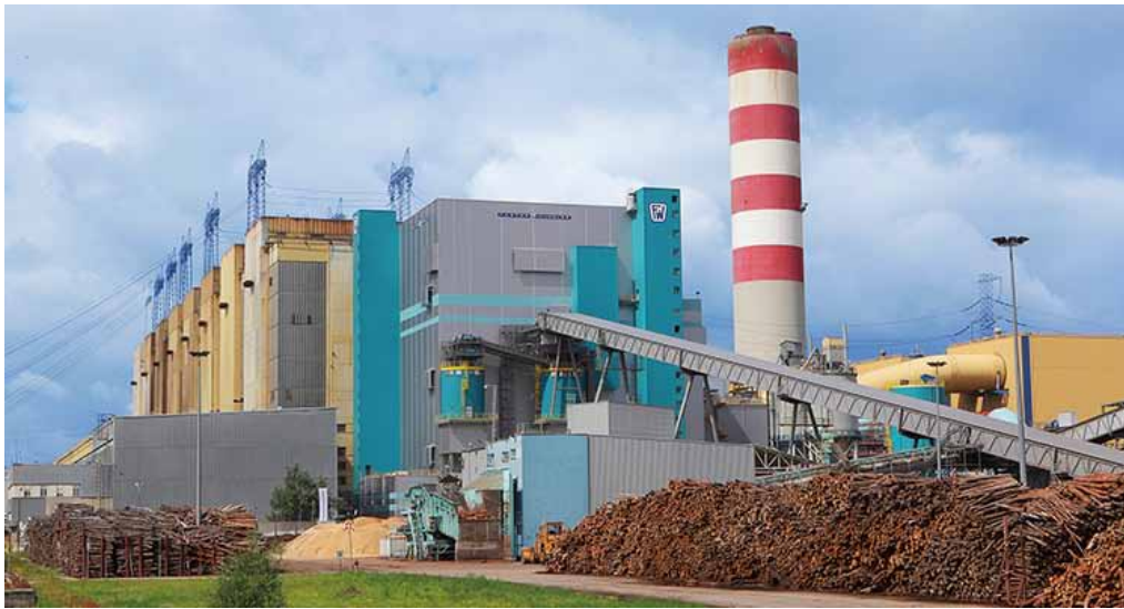
Figure 3 Polaniec Power Station (205MWe, 158.3/135.1 kg/s, 127.5/19.5 bar (a), 535/535 °C) supplies over 200 MWe of renewable power to Poland's power grid since 2012. The plant features SFW's state of the art advanced Bio-CFB boiler utilizing cutting edge design features and materials to efficiently and cleanly produce large scale power from a broad spectrum of wood biomass and difficult-to-burn agricultural crops and byproducts.
