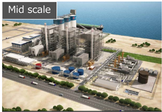
CFB boiler energy plants
