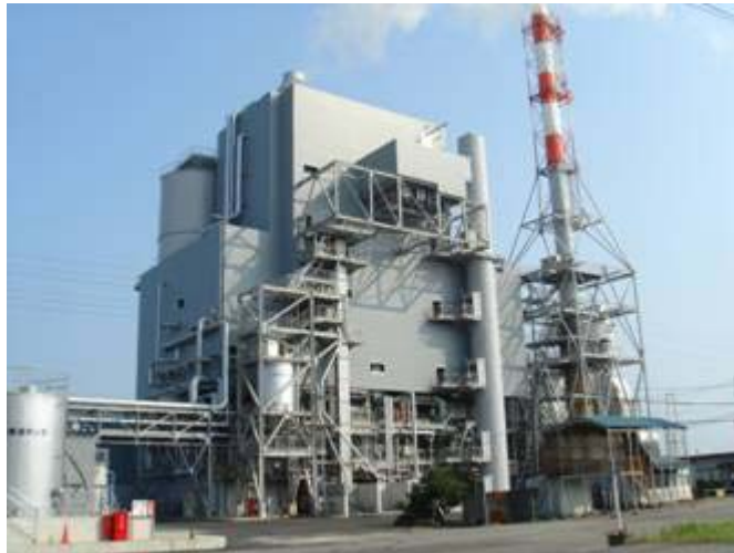
Use of CFB boilers contribute to reducing CO 2 emissions through effective utilization of energy resources and use of diversified fuels.
