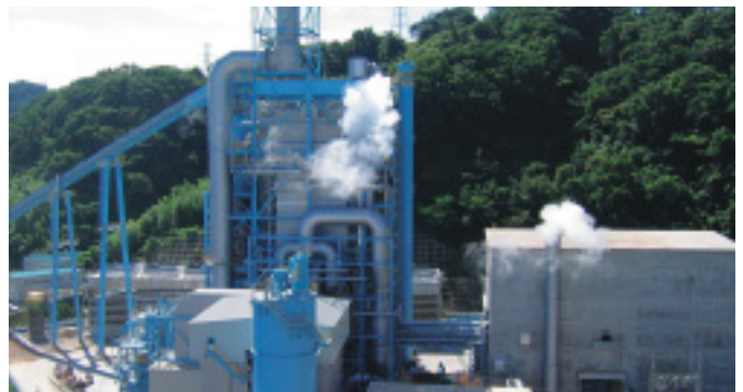
Tosa Power Inc. 167MW power plant
