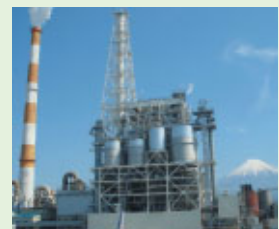
Nippon Paper / Fuji plant (under construction) Steam-generation capacity: 230t/h
