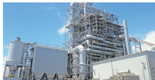
Biomass power generation plant (delivered to Mombetsu Biomass Electric Power)
