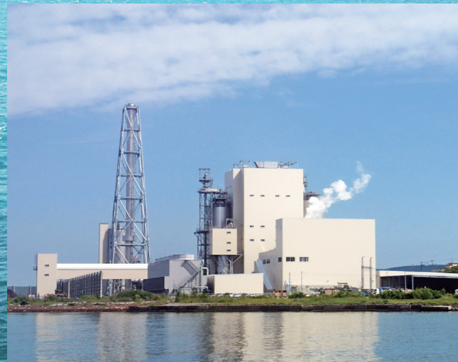
Biomass power generation plant (delivered to Summit Handa Power Corporation)
